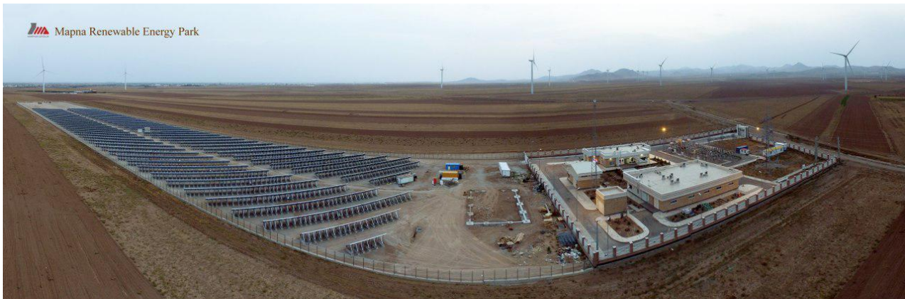
MAPNA's solar park is constructed beside its wind park.
